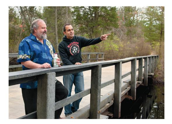
Nosker and graduate student Arya Tewatia on a New Jersey Pinelands bridge made of recycled plastic lumber.
